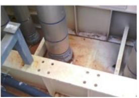
These images show roof penetration seals revealing a number of issues. Because of the close proximity of these joints to each other, if one fails it will cause the failure to spread to others.
